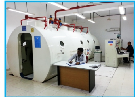
Six Man Chamber at GMH
